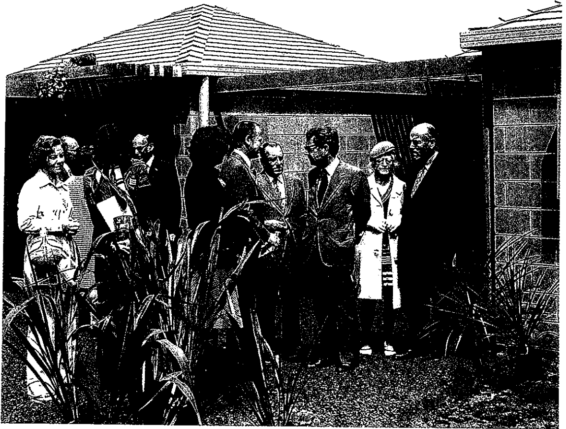
The official party inspecting Stage One units in 1975.
